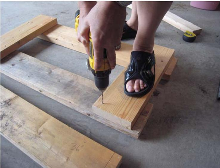
**3. Screw the crosspieces in place.** We used 2.5" screws, 4 on each end (16 total per side, 32 for both sides). We drilled holes before we drilled the screws.
